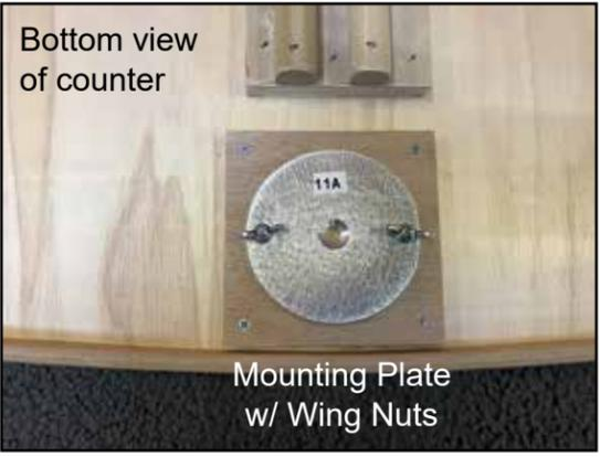
1) Mounting plate & wing nuts, in packed position.
